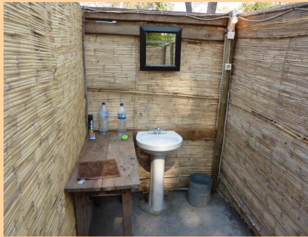
flush toilets & hot showers
